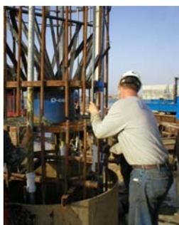
Installation of reinforcing cage with O-cell
